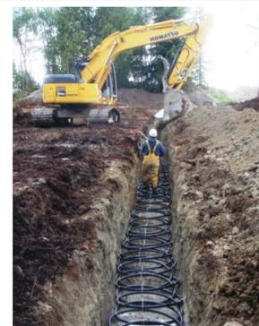
which are in turn connected to a heat pump inside the house. The heat pumps are similar to conventional ones. However, rather than draw off heat from the air, these pumps draw off heat from the fluid-filled pipes.
